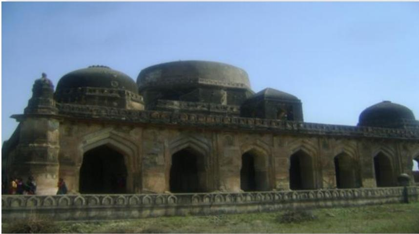
The Chaurasi Gumbaj is built of blocks of concrete set in lime mortar with style very closely with that of Lodi period. The whole building is divided like a chess board into eight line of piers and seven lines of open spaces, thus forming 64 piers all connected by twice 49 arches, with the 49 intervening spaces covered by flat roofs. In the middle, there are four piers omitted and the
